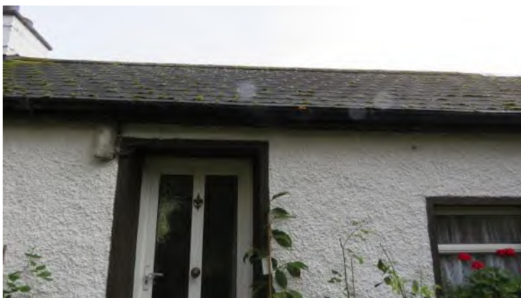
Photo 15 – close up of front elevation of roof of dwelling house
