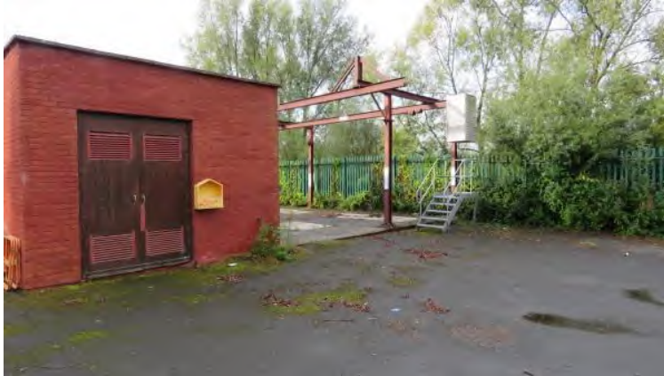
Photo 25 – small red brick building housing pumping equipment
