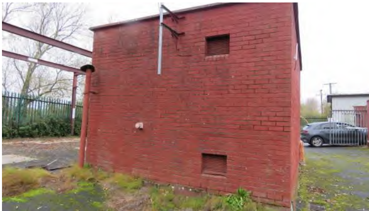
Photo 26 – rear of small red brick building housing pumping equipment
