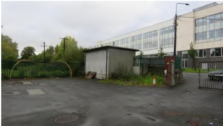
Photo 29 – small cement building at pumping station
