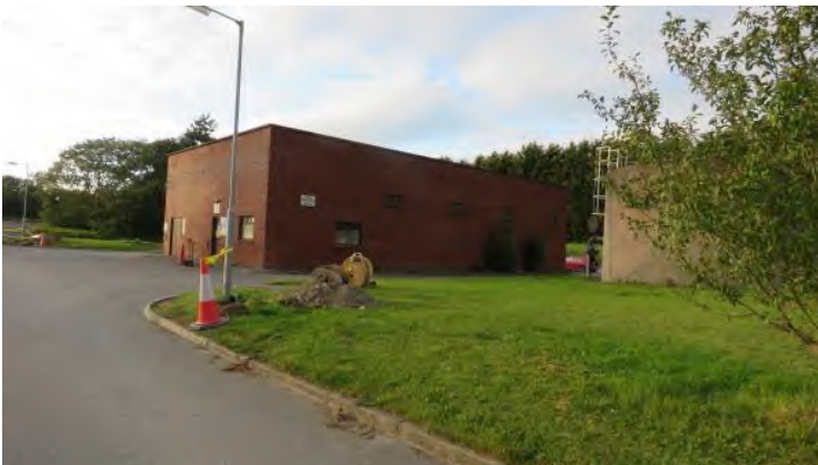
Photo 6 – large red brick in-flow building at north western corner of site
