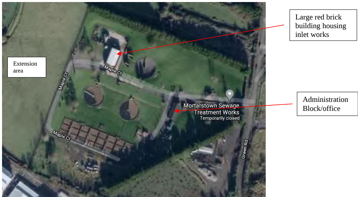
Figure 1 – aerial view of layout of Mortarstown Waste Water Treatment Plant
