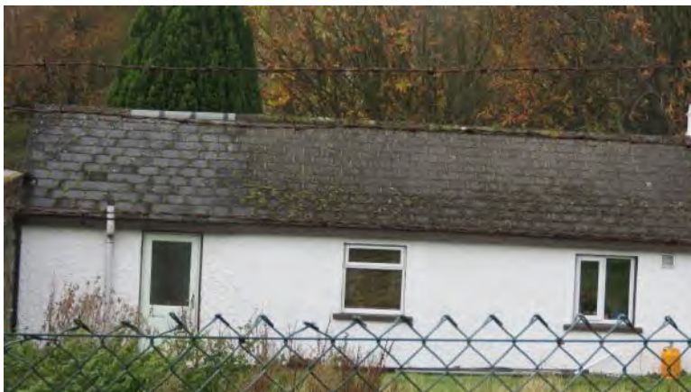
Photo 21 – Rear of dwelling house backing onto proposed extension area. Roof appears to have potential access points for bats
