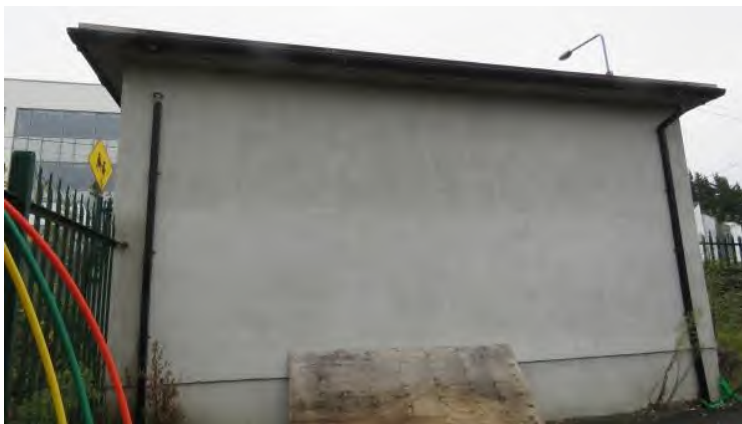
Photo 30 – no obvious roosting potential for bats in cement building
