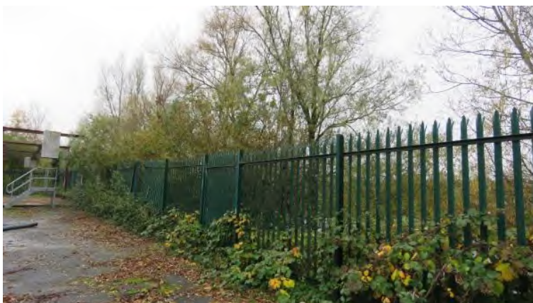
Photo 32 – Western boundary fence along River Barrow with semi mature willow along river banks
