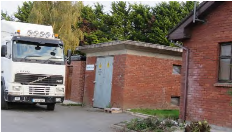
Photo 2 – red brick sheds to rear of administration building
