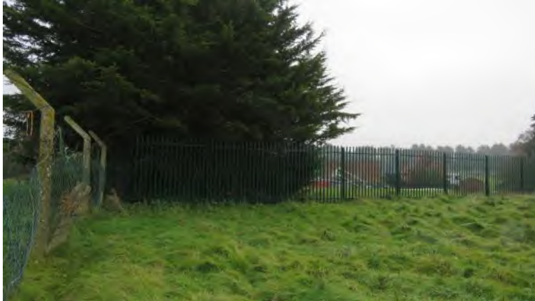
Photo 22 – boundary fence between existing Mortarstown site and proposed extension area
